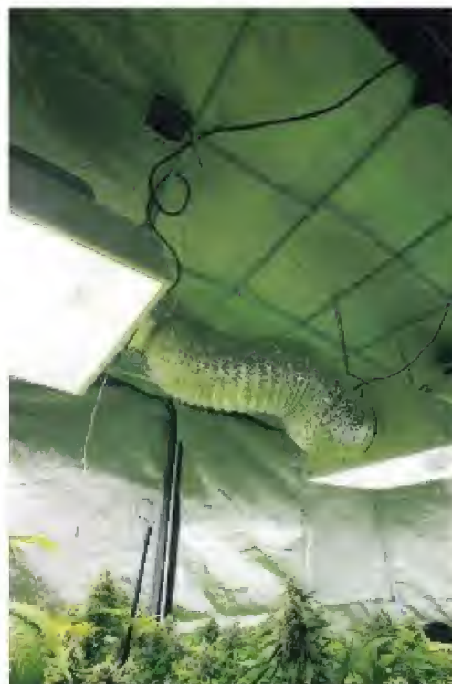
Inside, tents come ready-made for everything from lights to ducting to fan ports.
